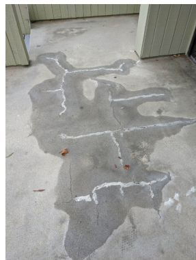
Example of the clubhouse deck surface in need of repair
