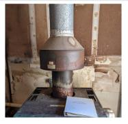
see in these pictures), which may have been due to improper storage of the muriatic acid and chlorine in the common space of the pump room.
