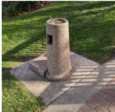
The existing stone aggregate drinking fountain that is being replaced
